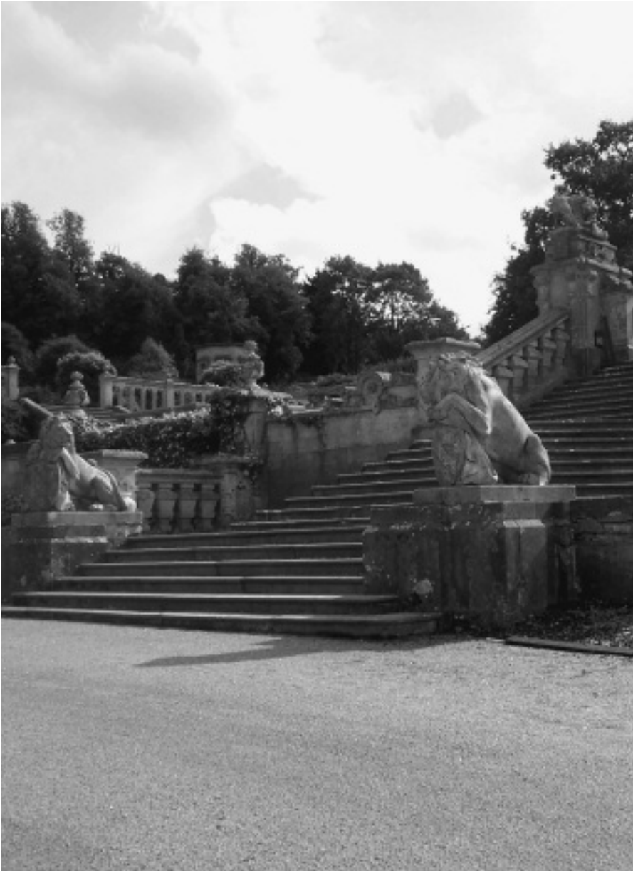
Steps to Garden off Front Circle
